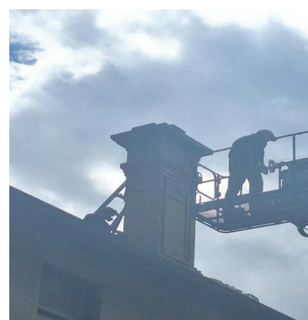
Crew making repairs to the chimney so we can use the fireplace this winter.
